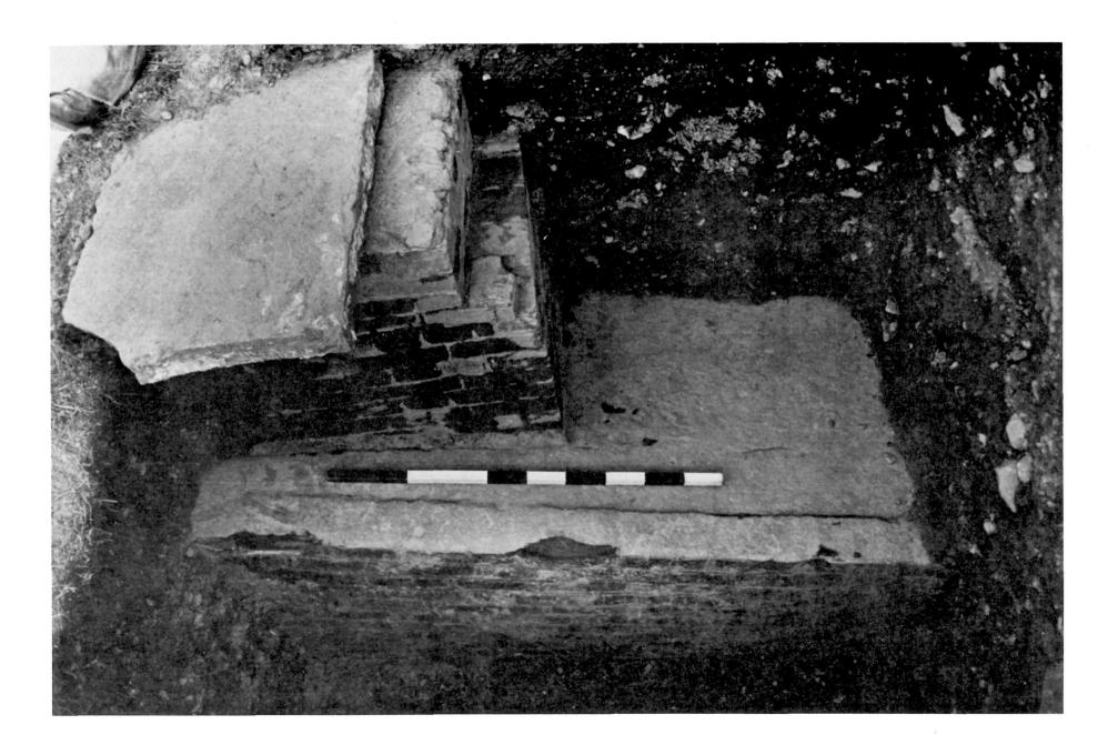
Overview of sub-operation 2B23T on right face of the southeast salient which exposed the foundation for the smoothbore emplacement and its pivot location.
