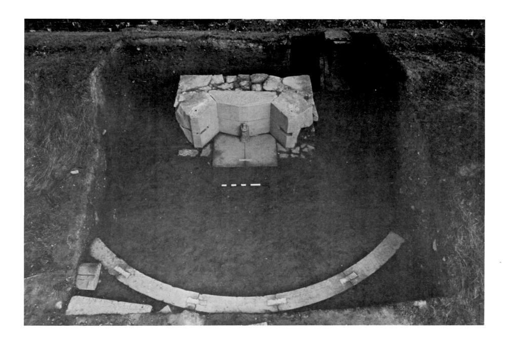
14 Cast iron pivot  $\underline{\text{in situ}}$  with forge welded wrought iron axis. Note the extremely narrow joints with mortar between the segments of the granite behind the pivot. (Scale 1.0 m)
