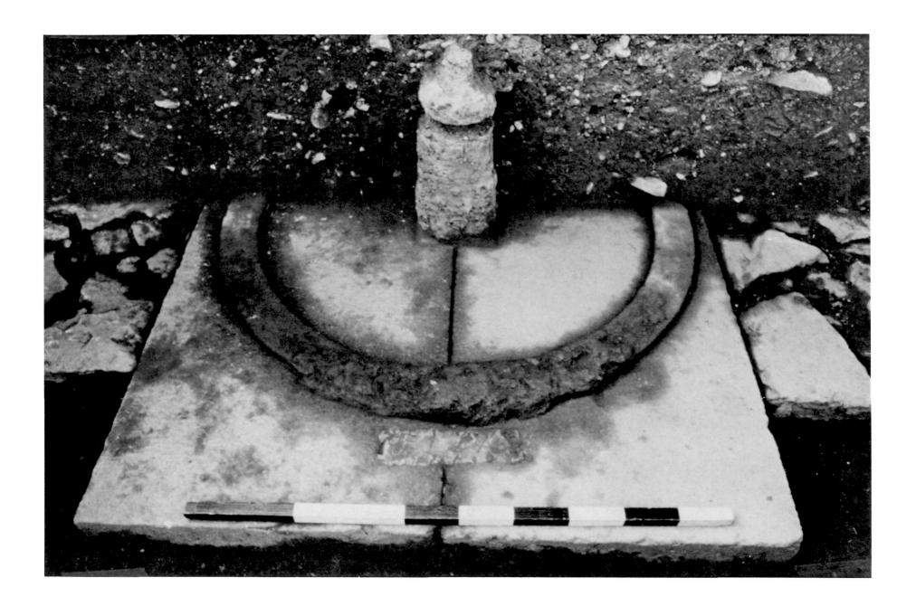
23 Excavated base for chimney in sub-operation 2B32F on the right face of the NWDB. Note the seyssel asphalt water-proofing on the flue below the chimney. (Scale 1.0 m)
