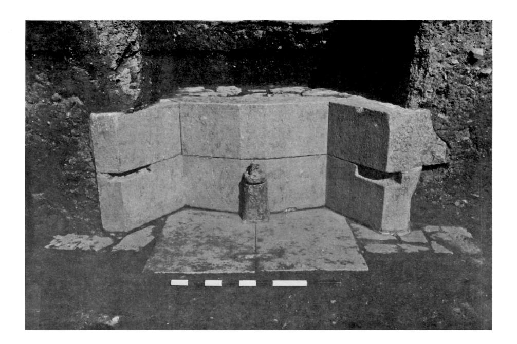
12 Front view of excavated 32-pound smoothbore emplacement on the right face of the northwest demi-bastion. Note the two slots cut into the two lower segments of granite, especially the incomplete slot on the left wing. (Scale 1.0 m)
